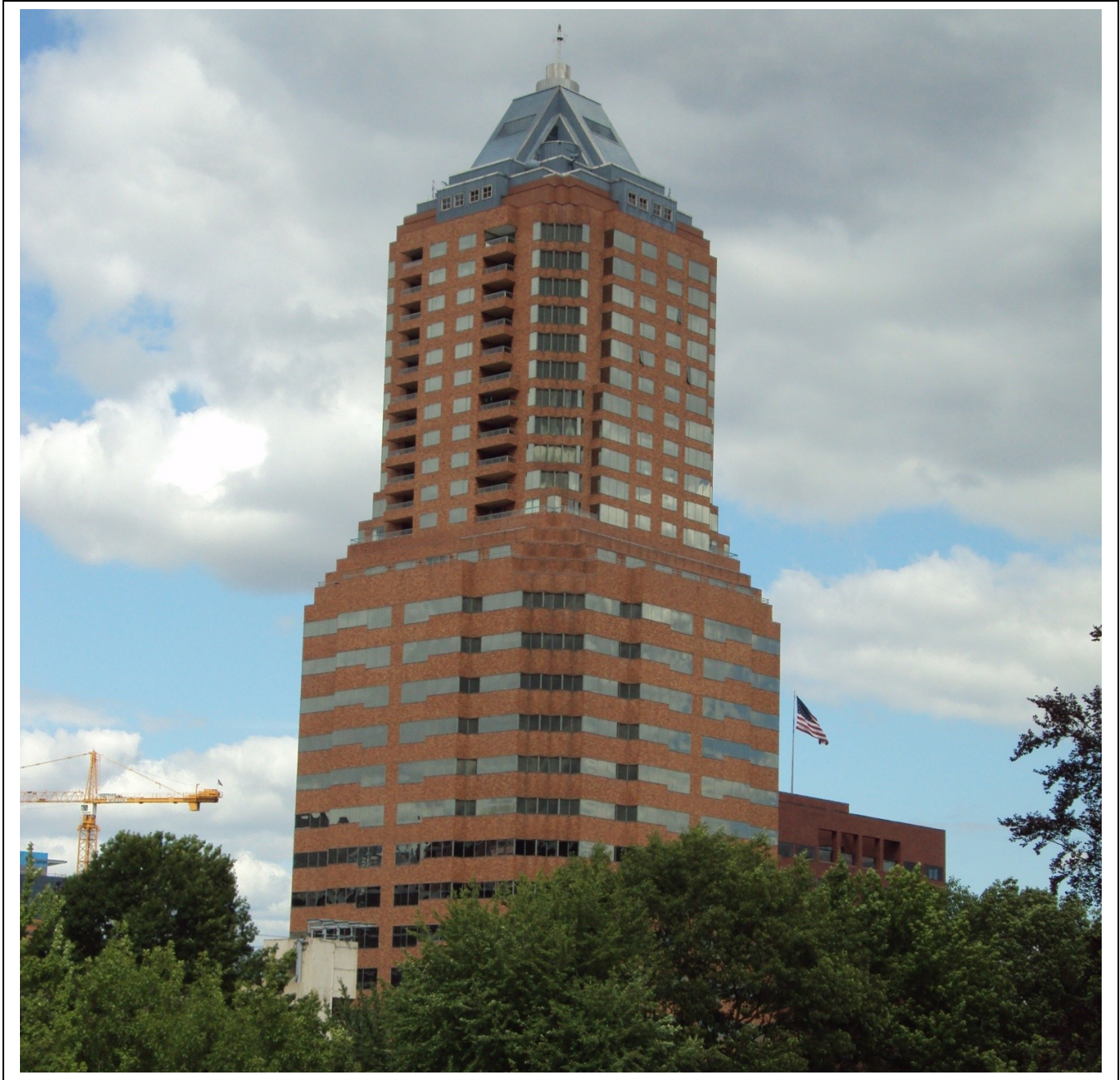
KOIN Tower - Downtown Portland Oregon
