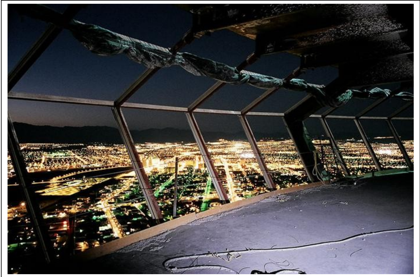
View from Stratosphere during construction
